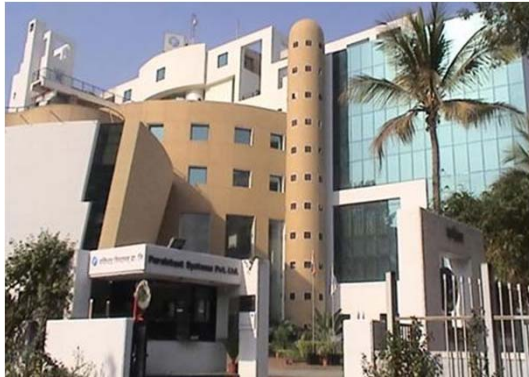
Senapati Bapat Road, Pune (operational)
