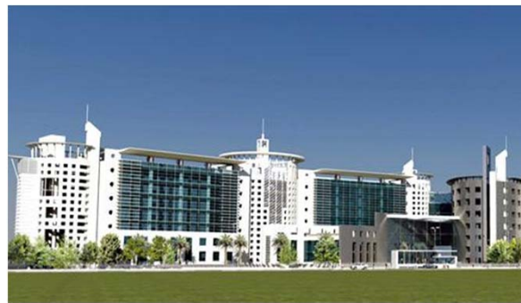
Under construction (artist impression)
