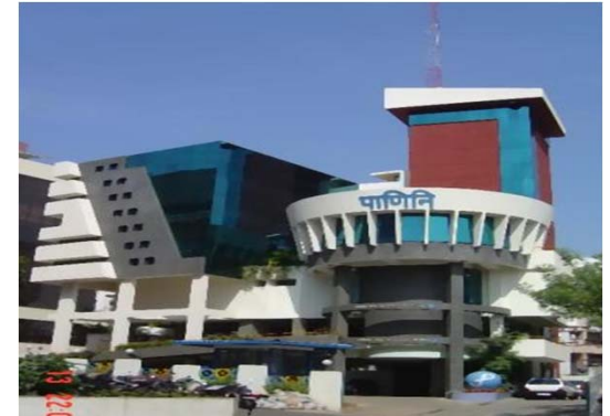
Senapati Bapat Road, Pune (operational)
