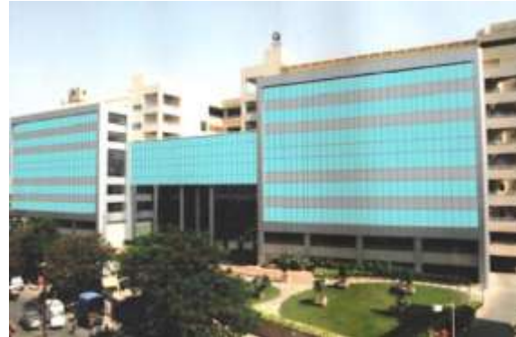
Karve Road, Pune (operational)
